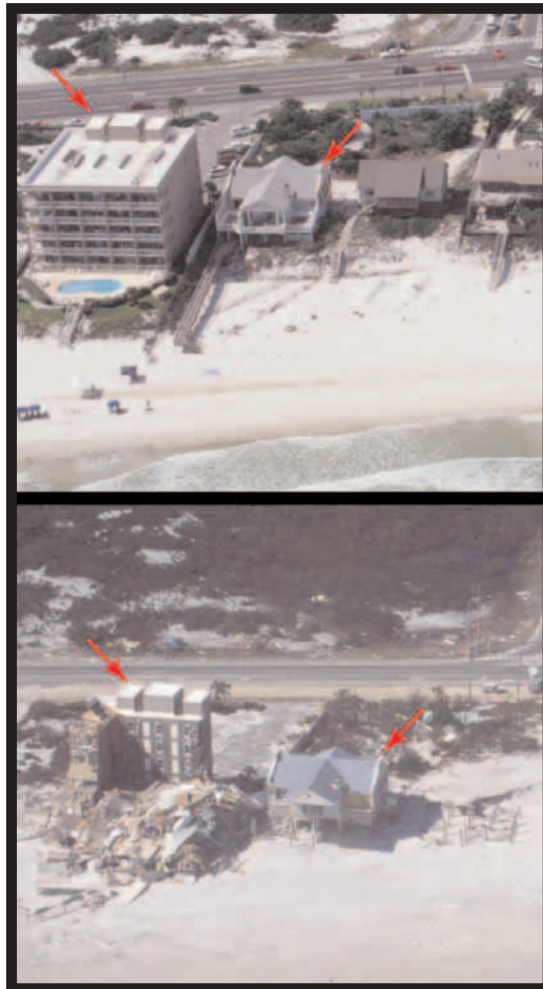
Orange Beach, AL before and after Hurricane Ivan
