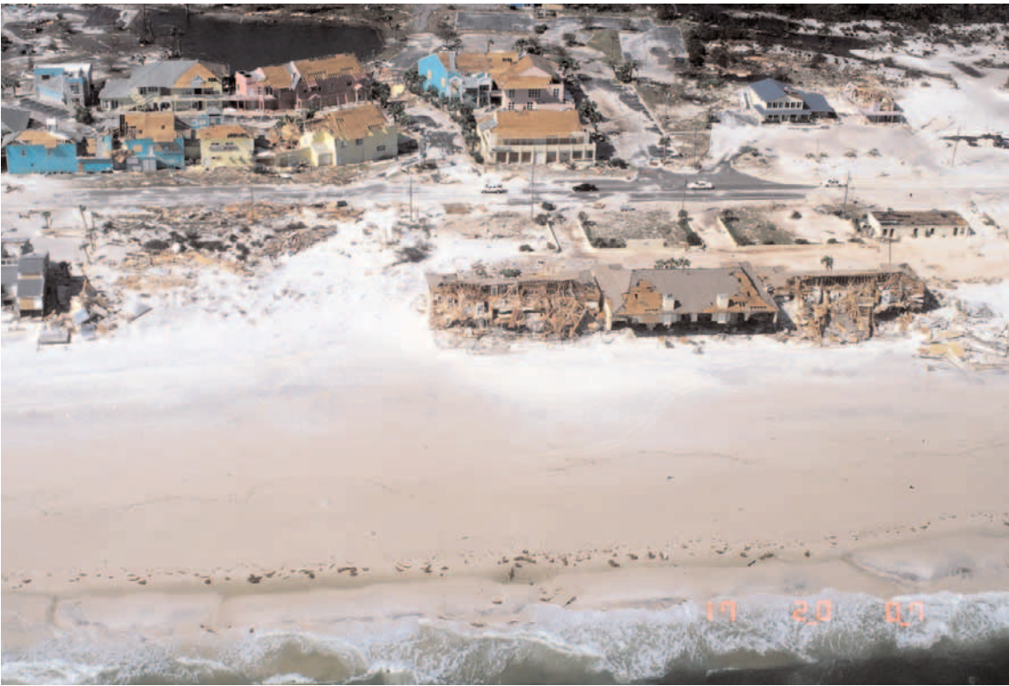
Orange Beach, AL after Hurricane Ivan
