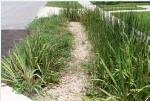
Low-impact development and green infrastructure such as bioswales (pictured) can help ease the burden on the aging stormwater drainage system. Photo: GRN.
